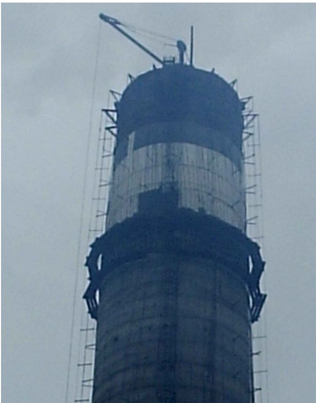
Fig. 2. Shoring the stem of H=60 m chimney of Magnitogorsk Sintering Plant
